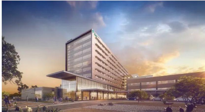
*In this rendering of the Phoenix-based Valleywise Health Medical Center replacement hospital, the bed tower is positioned with patient rooms facing east and west, requiring special consideration for solar heat gain, daylighting and glare. Courtesy: EYP Architecture & Engineering and Cunningham Group*
