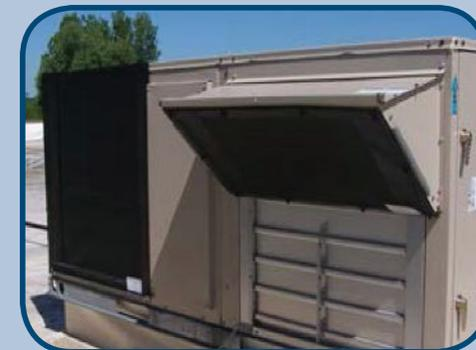
**Snow Stopper™ Screens Mount inside or outside louvers and on rooftop air handling units for a snow barrier at point of entry.**
