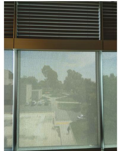
The lower shade has a 3% openness that provides views and outdoor connection while shielding the occupant from glare and heat. Credit: New Buildings Institute
