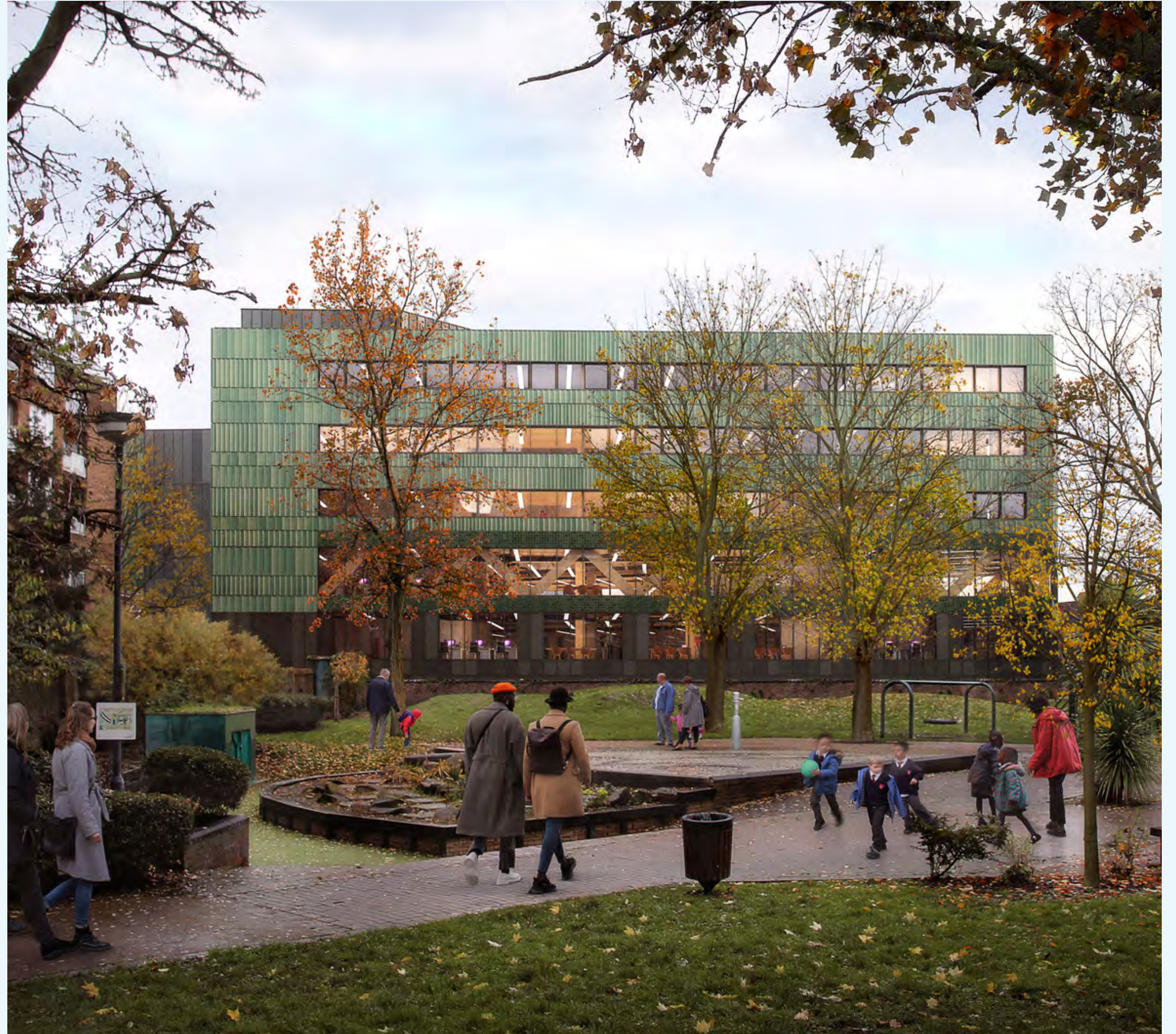
Paradise is a proposed office building that will be built with crosslaminated timber and aims to be carbon negative for at least 60 years. By FCBstudios.
