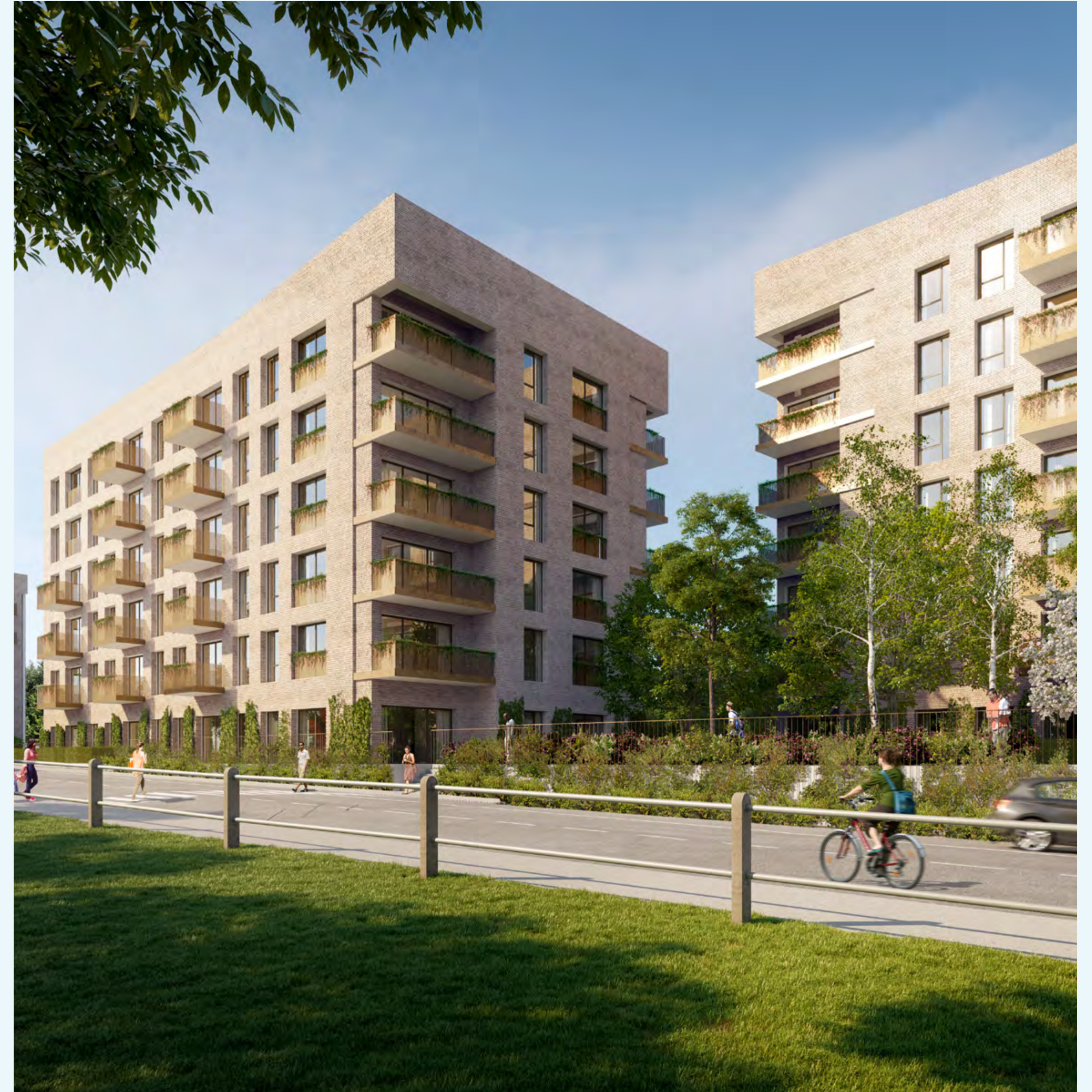
Land at High Barnet station is a zero emissions development transforming a car park into housing. By Scott Brownrigg for TfL and Taylor Wimpey.
