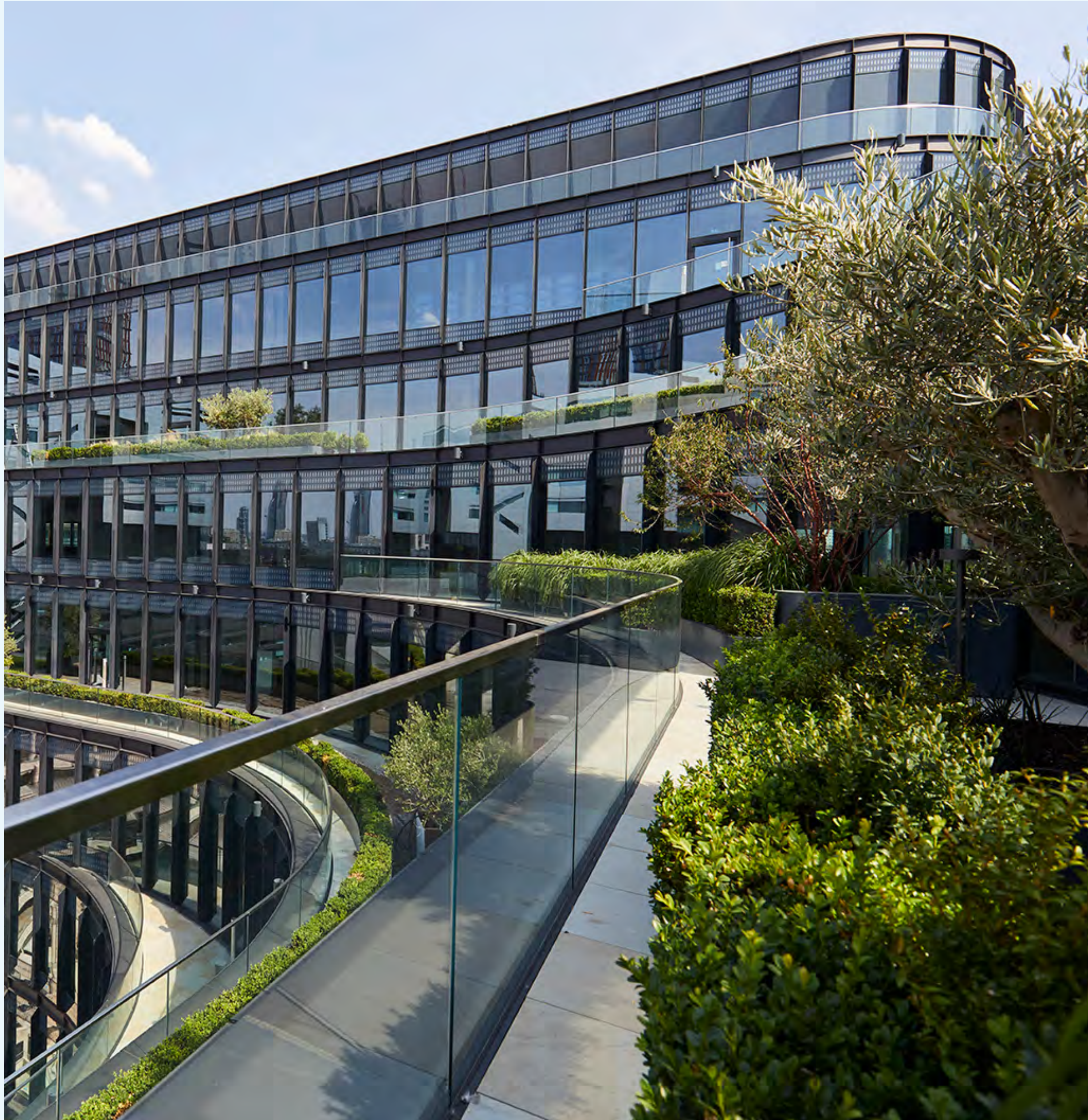
100 Liverpool Street is a converted 1980's office building targeting BREEAM Outstanding, with over 49% of retained and reused concrete. By Hopkins Architects for British Land.
