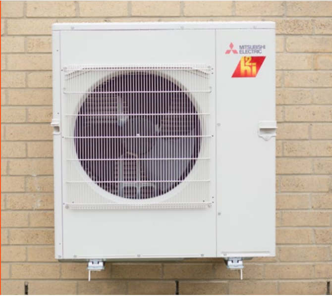
Figure 2: Outdoor compressor unit of heat pump
