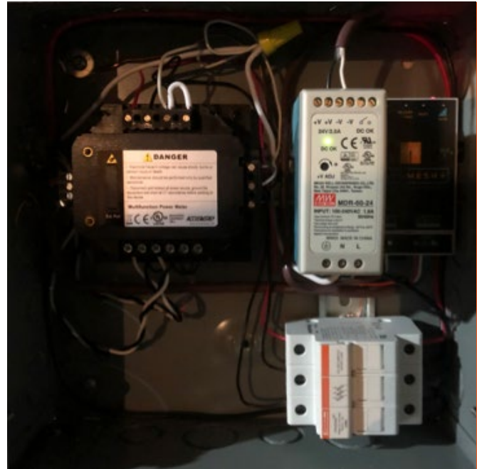
Figure 3: Electricity metering.
