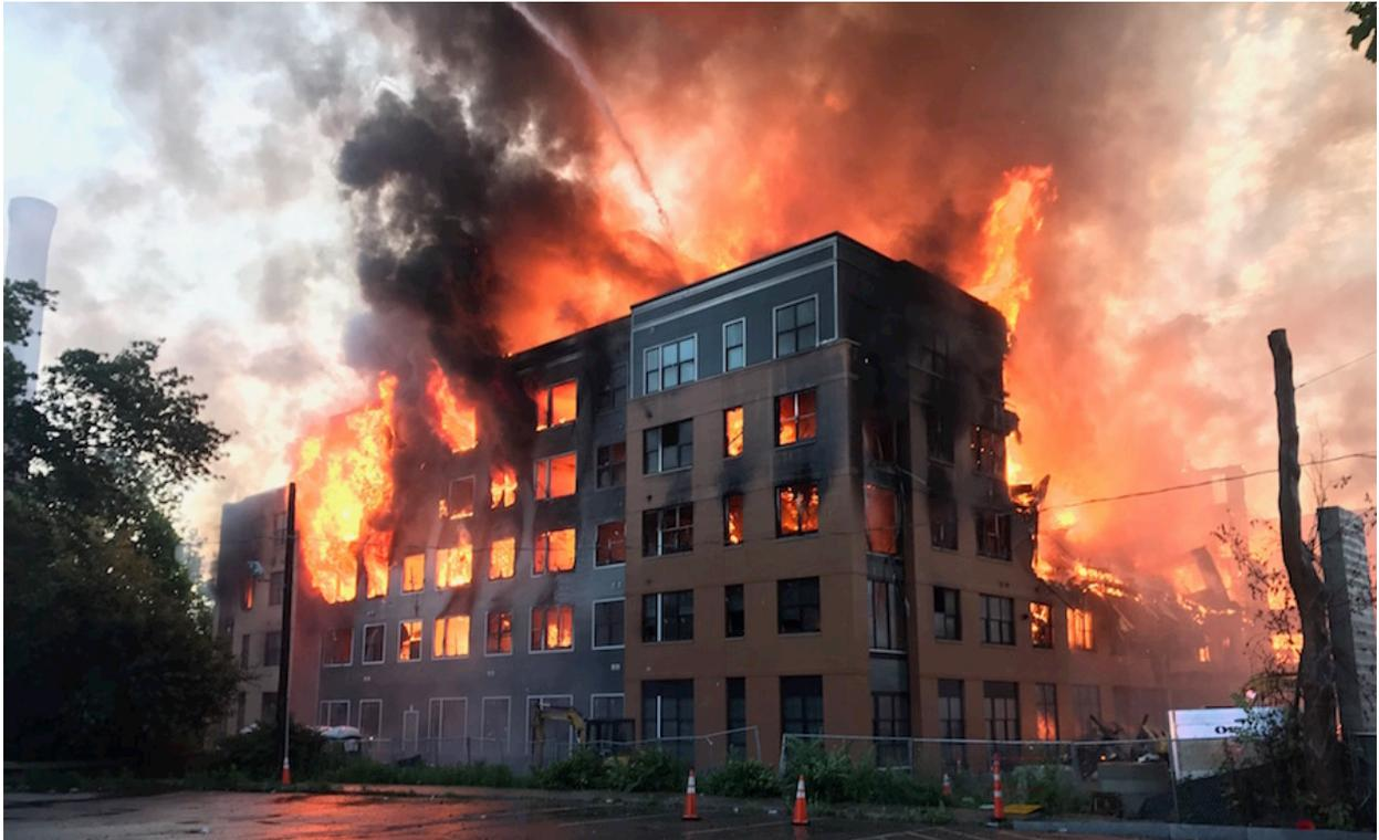
Figure 3.10 Fire in Timber Frame Apartment Building Under Construction (Source: Captain John Bonadio, Waltham Fire Department, as published at <https://www.enr.com/articles/42484-what-local-officials-want-to-do-about-wood-frame-building-fires-in-massachusetts> (last accessed September 2020), Courtesy of Waltham, Massachusetts Fire Department)
