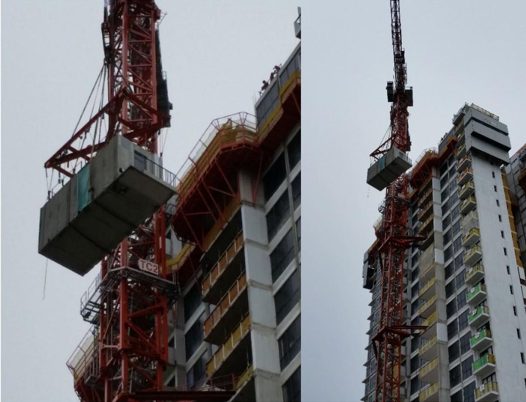
Figure 4.5 Precast Concrete Modular High-rise Construction in Singapore – Module Being Lifted into Place by Crane (Source: Brian Meacham)
