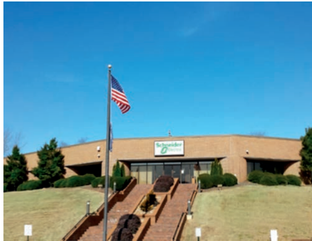
Figure 3-16 Schneider Electric’s Seneca Manufacturing Facility
