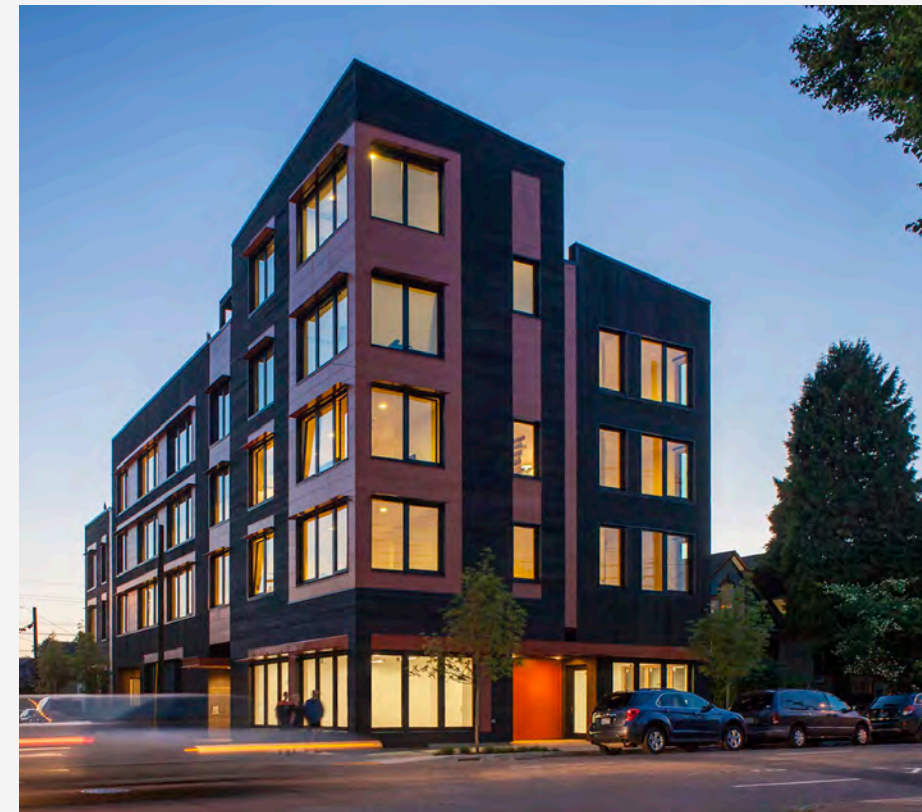
Top Kiln Apartments, Portland OR Bottom 100 Pike, Seattle, WA
