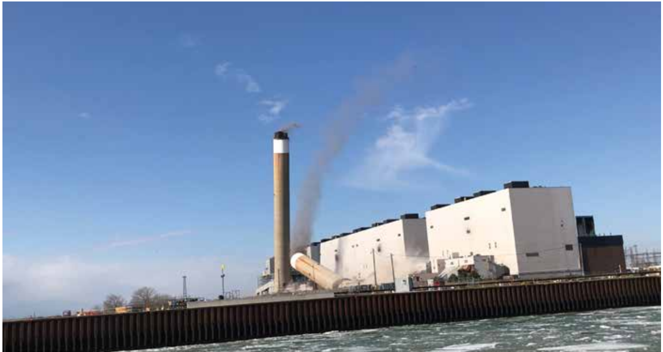
Bringing down the last two stacks at Nanticoke generating station (28 February 2018).
