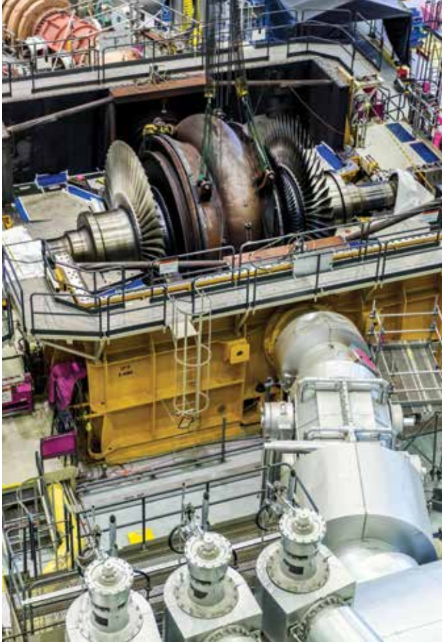
Turbine removal in the Darlington refurbishment. Source: Ontario Power Generation.
