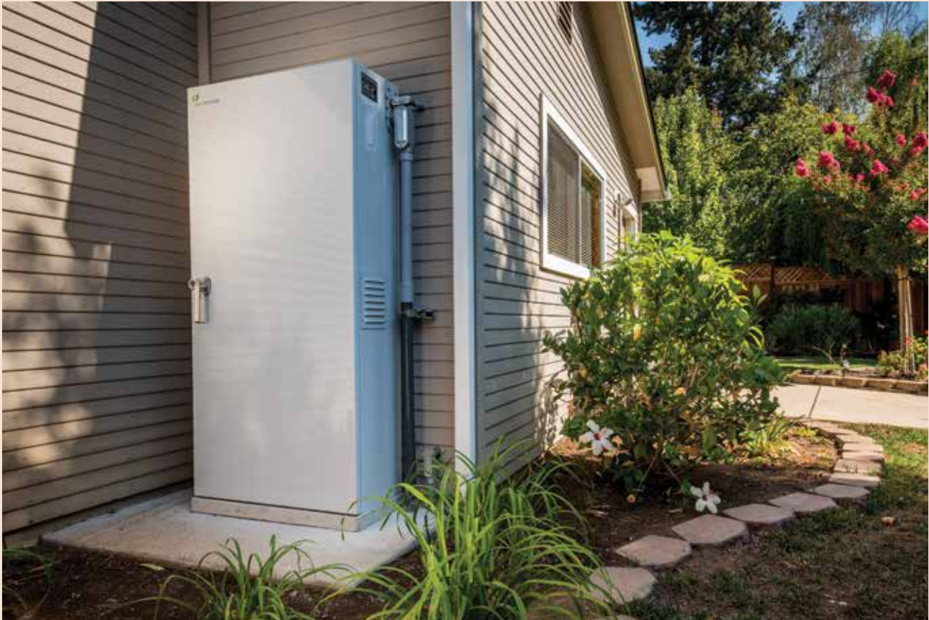
Sunverge's residential solar electricity battery storage system used by Alectra Utilities in their Power.House demonstration project.
