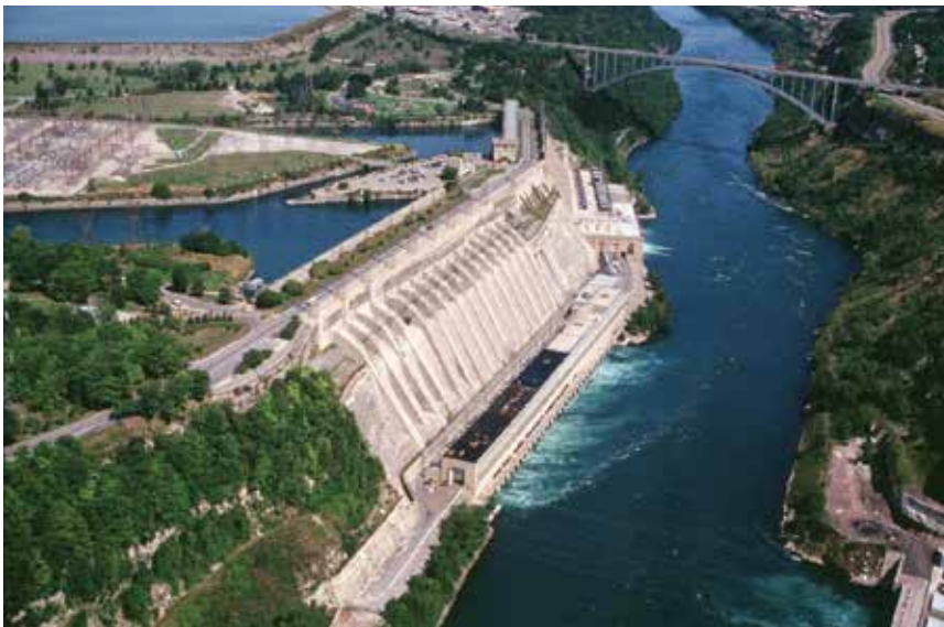
Sir Adam Beck Generating station, with the pumped storage hydro reservoir on the top left, Niagara Falls, Ontario.
