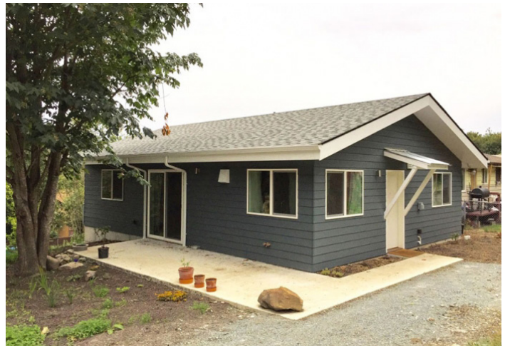
Zero Energy Ready Home in Seattle, WA.
