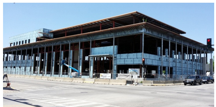
Air-sealing a new construction building in China.
