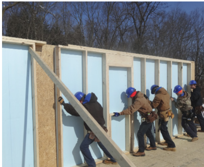
Field installation of extended plate and beam wall system.
