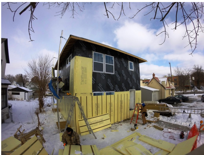
Field testing a moisture-managed, solid panel wall system.
