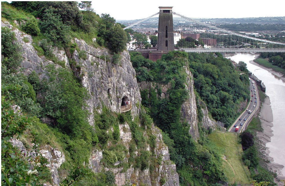
A view of Clifton Suspension Bridge—an illustration of the challenging RF landscape that the city has to accommodate
