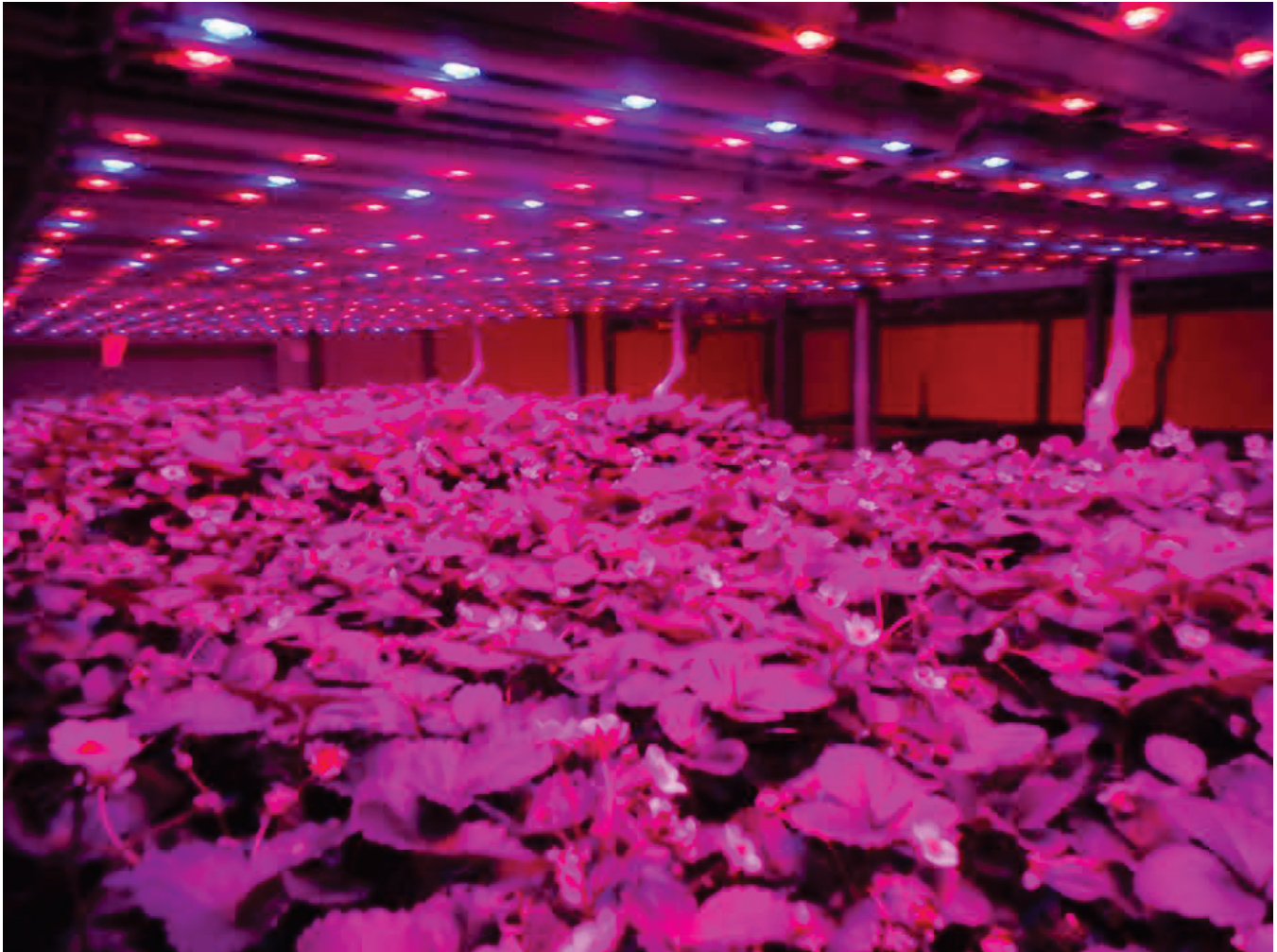
FIGURE 4.6 Some plants grow well under lighting that would not appeal to humans and has very poor luminous efficacy as expressed in lumens per watt. SOURCE: Neil Mattson, Cornell University, “LED Lighting for Plant Applications,” presentation to the committee, February 24, 2016.
