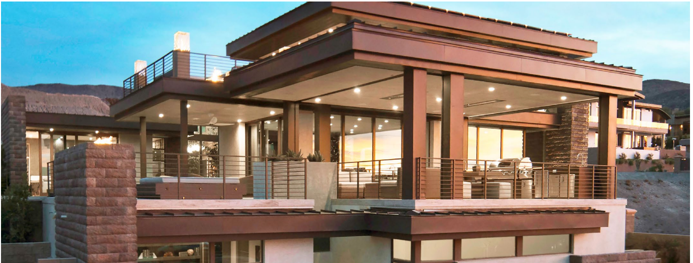
The 2016 New American Home has a fully encapsulated building—walls at R-33 and R-58 in the roof.
